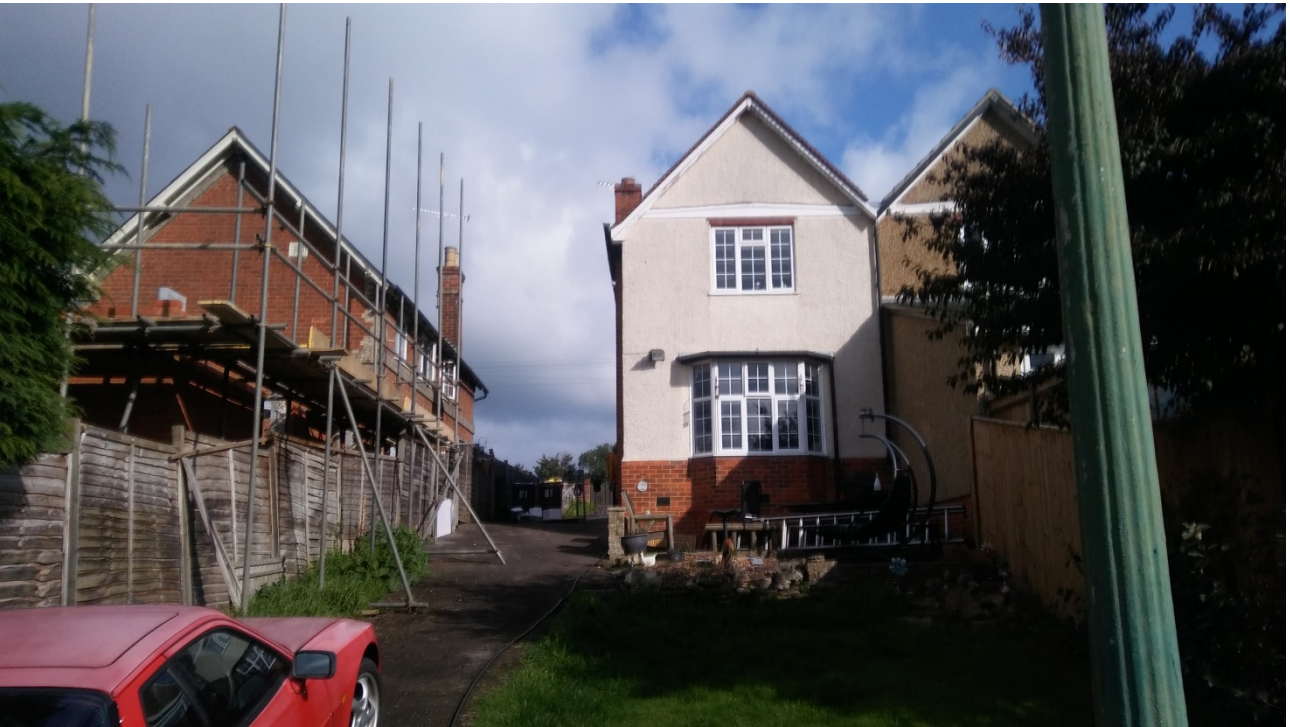
Photo taken from garden of 81 Henley Road (N.B. this was taken during withdrawn application 171302, when the ground floor extension was still under construction)
